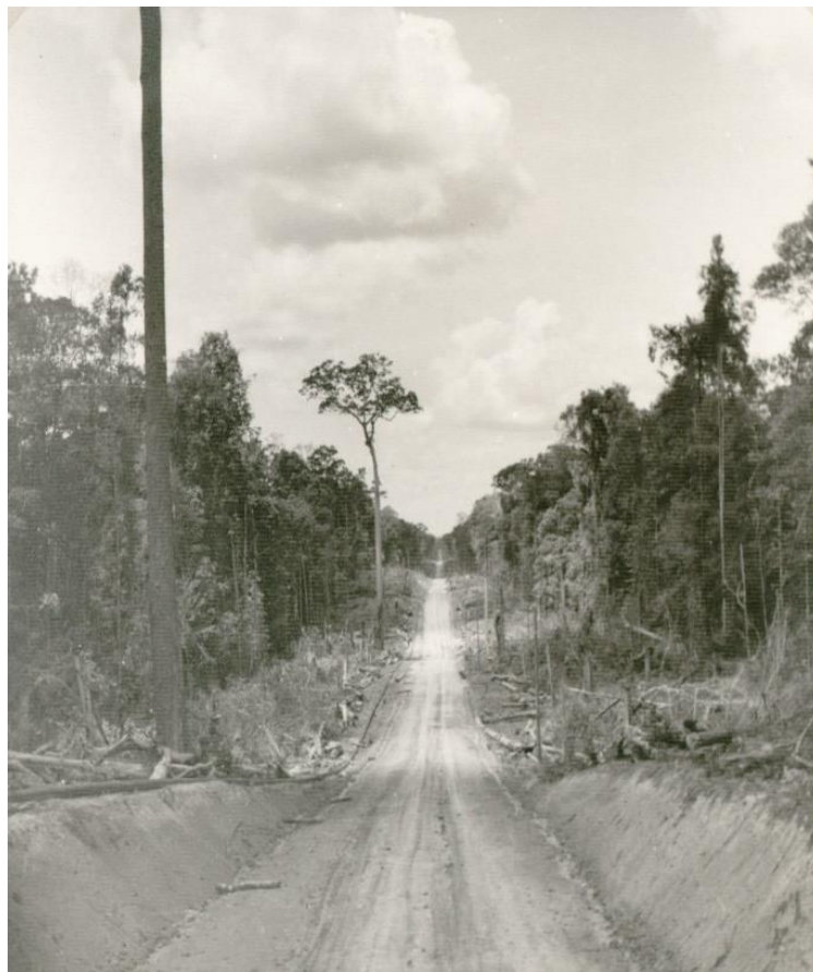
Image 4, Finished Road, Between Jambi and Palembang.
