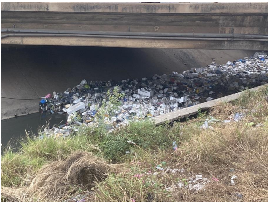
These pictures depict the current situation in Accra regarding SUP waste that blocks drainage systems, causing flooding. Most of the waste in the gutters is plastic.
