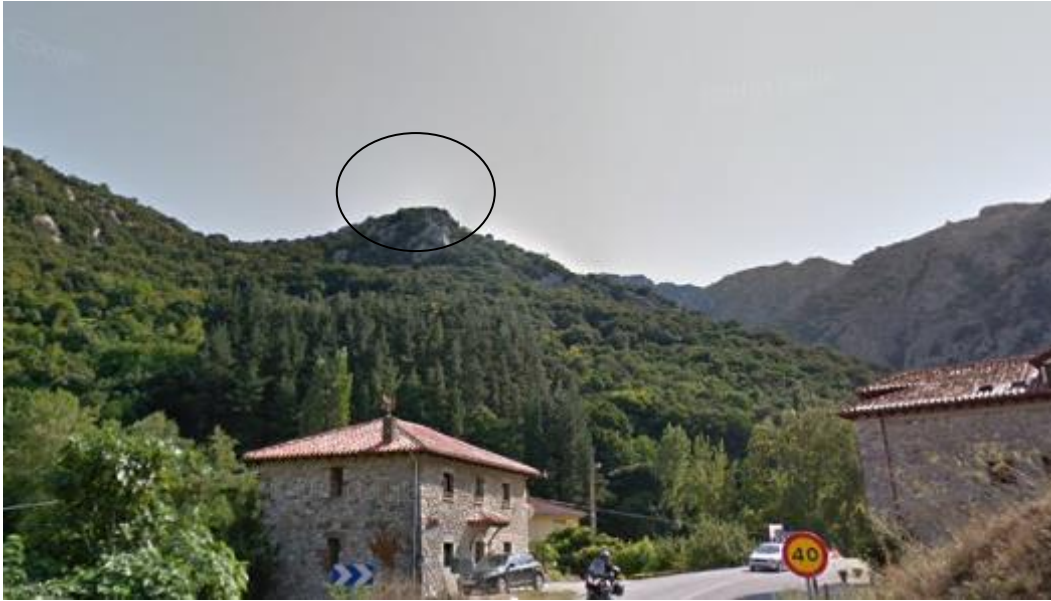
Figure 9. View of Torre Tevirde from Casa rural El Agero
