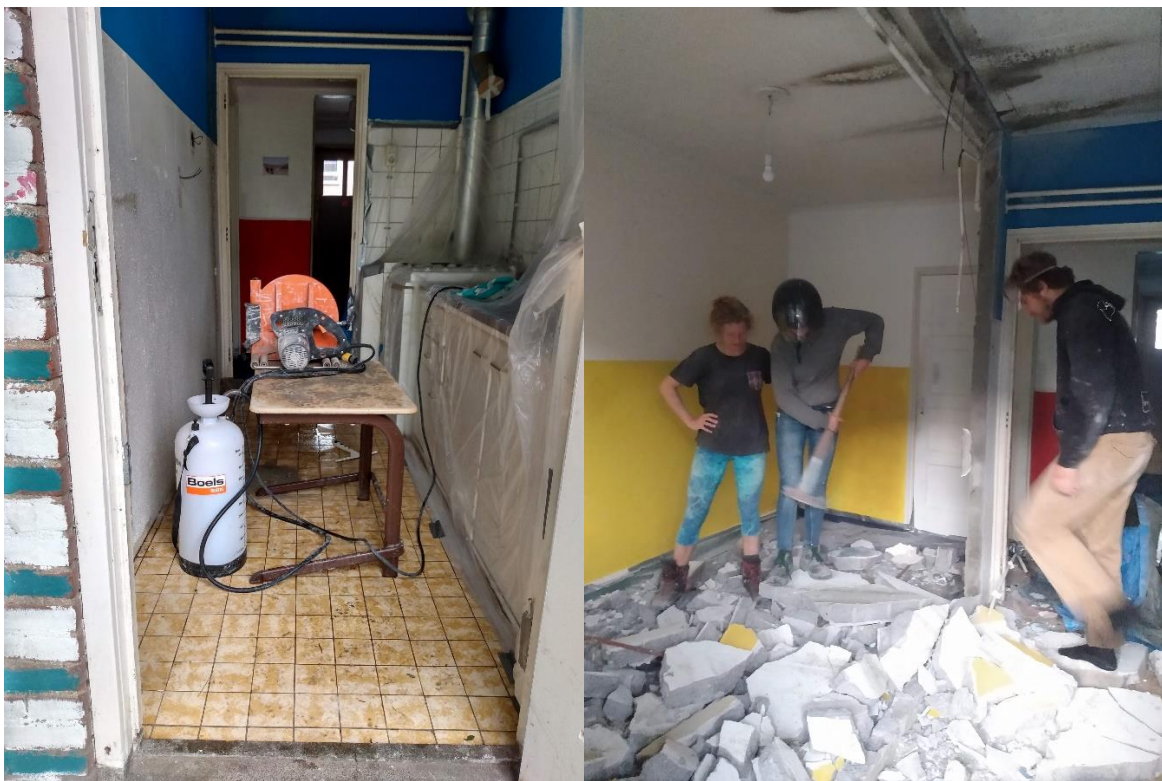
Figure 28 & 29 The wall saw. The kitchen wall in pieces.
