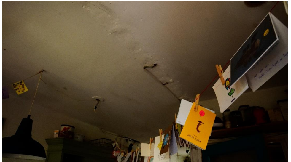
Figure 31 On the ceiling traces of the wall that used to separate the kitchen from another small room. Still by author.
