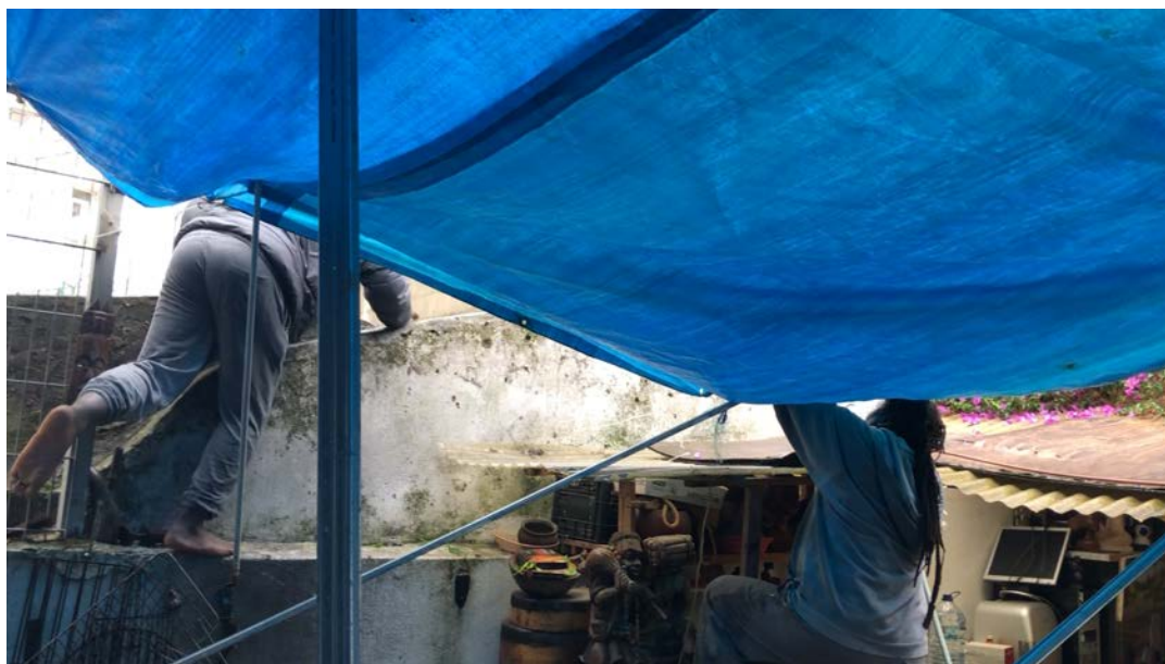
Note. Own work (Photo taken on the 24 th of December 2021)
