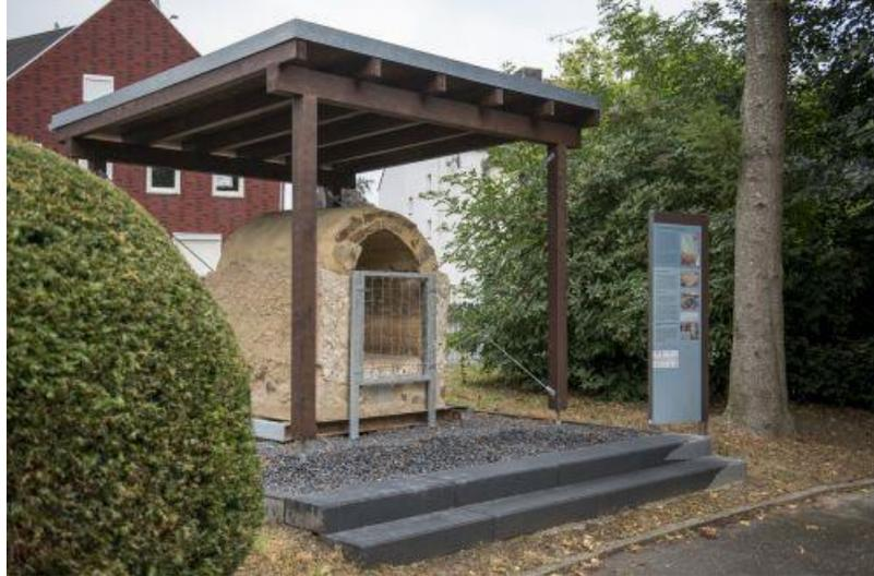
**Figure 14.** A section of the Roman pipeline in Würselen (Claßen and Vollmer-Köning 2021, 7).
