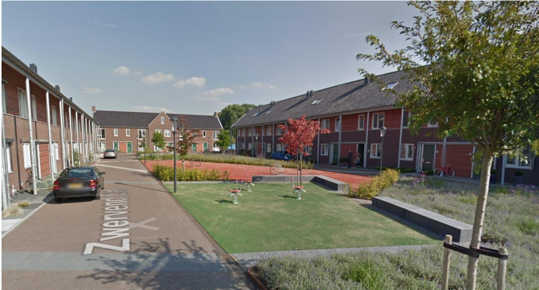
Figure 12. One of the outlines functioning as gathering place in the courtyard Zwervend Erf (Google Street View).
