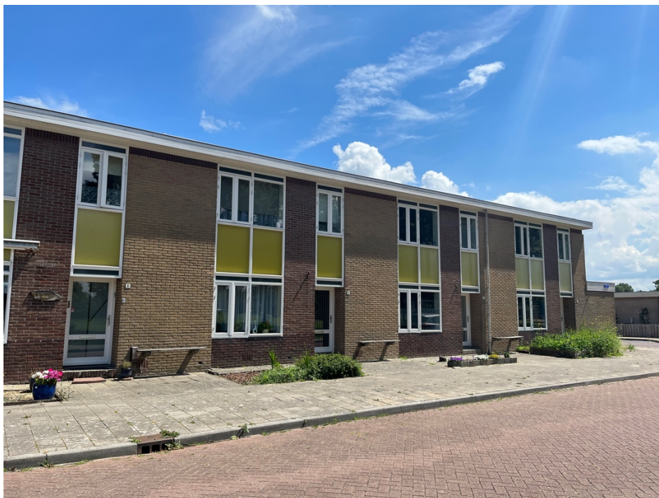
Figure 3.17: Houses designed by Rietveld in Nagele. The houses contain a particular kind of colored and armed glass which was a new building material adopted by the modernist architects during the 1950s.
