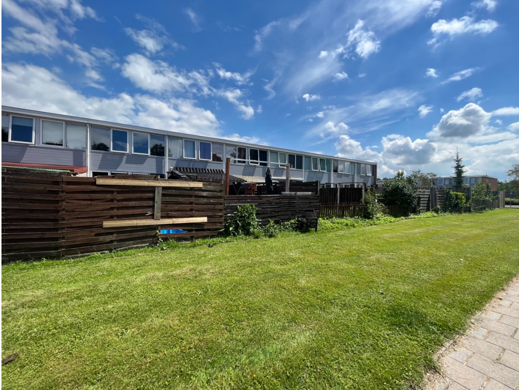
Figure 3.18: Houses show visible signs of deferred maintenance..
