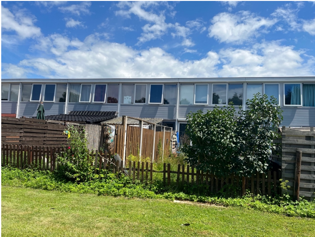
Figure 3.19: Houses show visible signs of deferred maintenance.
