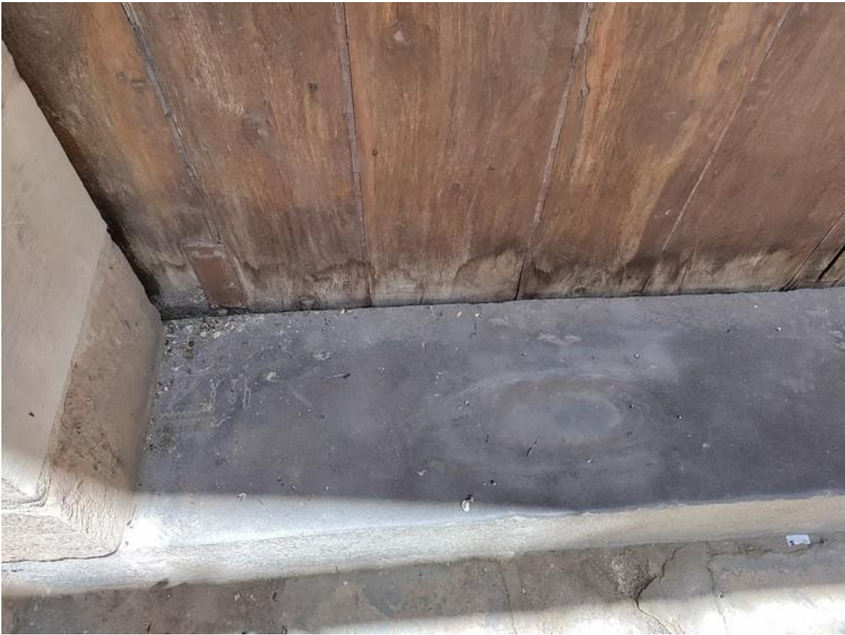
Figure 4. The left block of the threshold showing hieroglyphs at the main entrance of the Aqsunqur Mosque (1346 AD). The photo is taken from the road (PHOTO BY THE AUTHOR).
