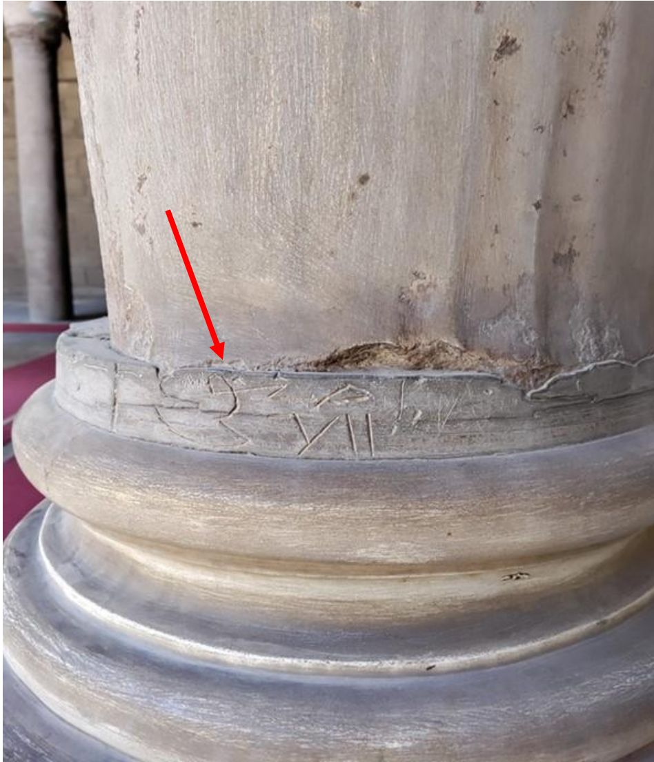
Figure 8. Example of a metal band with graffiti (red arrow) that attaches the base to column in the Mosque of Sultan Al-Nasir Muhammad (1318 AD) (PHOTO BY THE AUTHOR).
