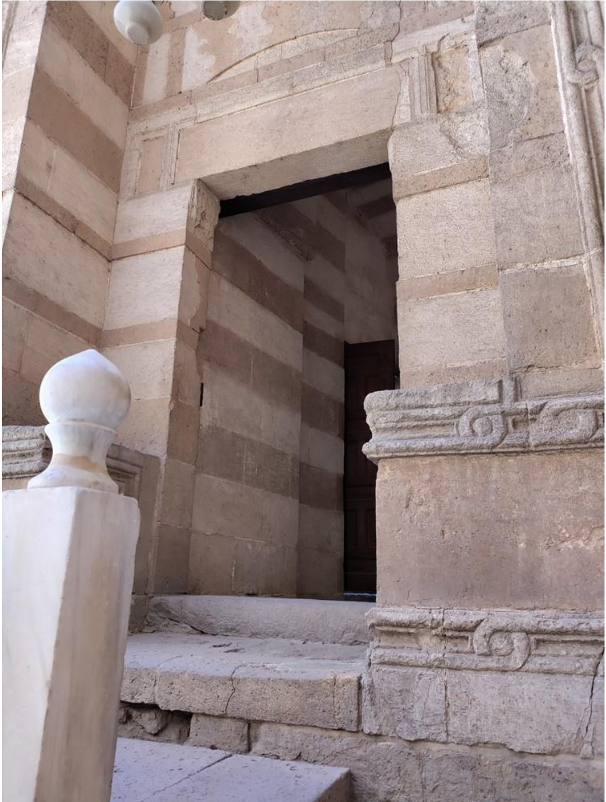
Figure 6. Entrance of the Funerary Mosque of Khayrbak (1502 AD). Photo is taken in the funerary complex from the outside of the mosque (PHOTO BY THE AUTHOR).
