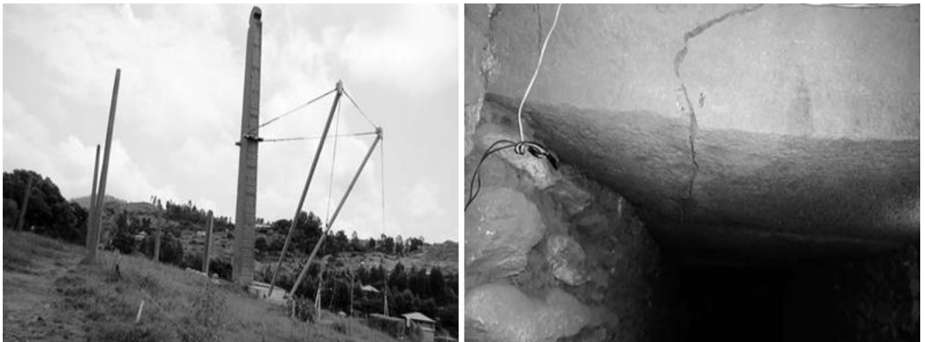
Fig. 72: Cracks in the slabs supporting the doorway to Mausoleum (Hagos, 2018; 301) Destabilized Stele 3 and current support system in place (Hagos, 2018; 302)
