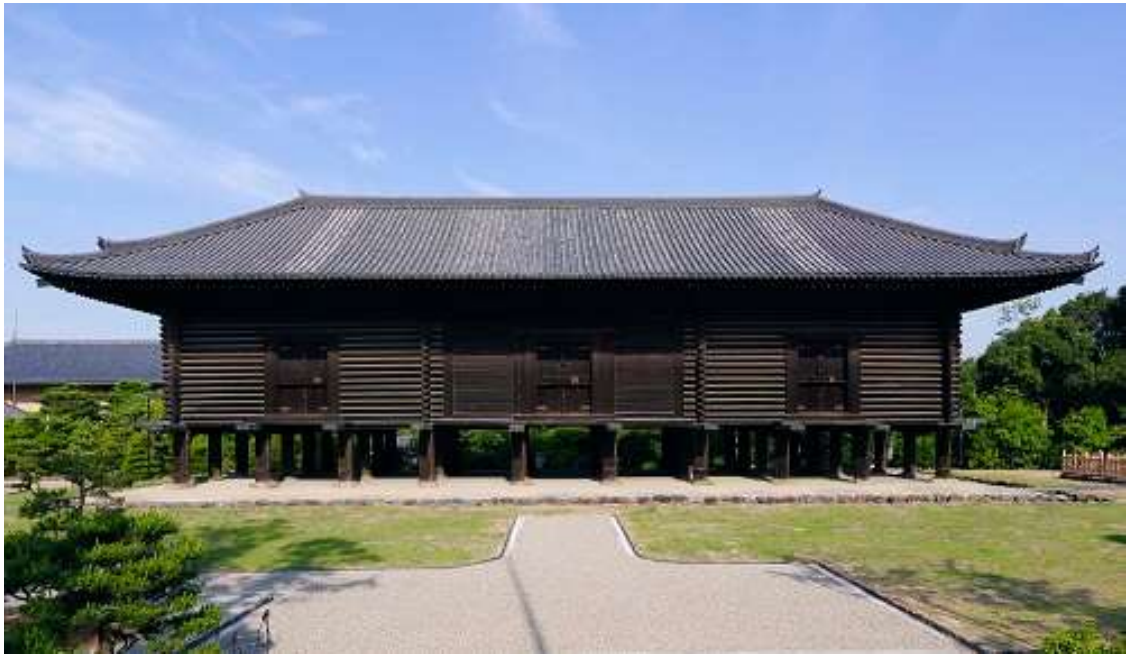
Figure 5 – Picture of the Shōsōin Repository, the historical treasure house of the Tōdaiji temple in Nara. Estimated to have been built during the second half of the 8 th century.
