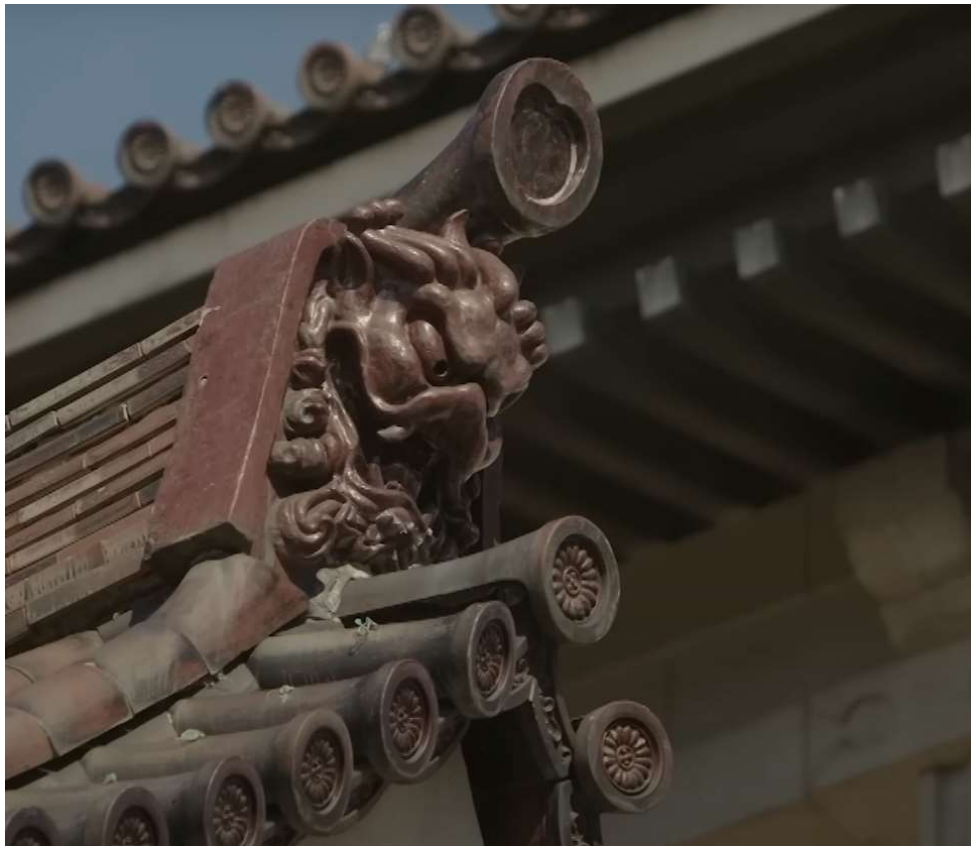
Figure 16 – An onigawara roof tile. Detail of the roof of the Honkan.
