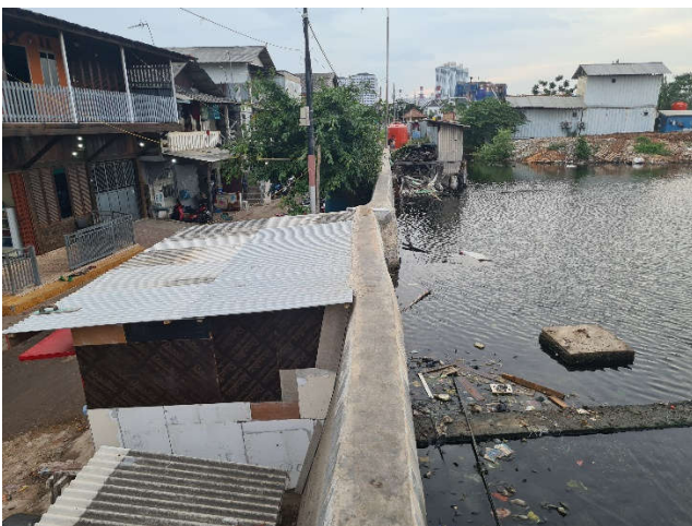
Figure 4. The seawall in front of Kampung Gedung Pompa.
