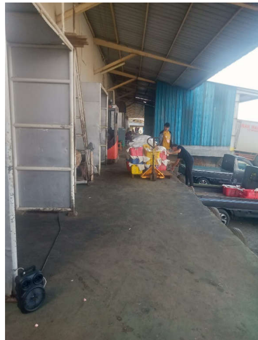
Figure 37. A kastorit building in Muara Baru. (Photo by research participant)
