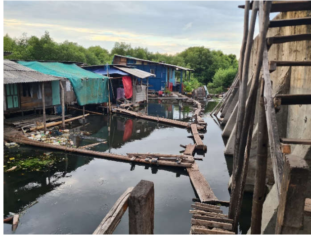
Figure 8. Houses built on flooded positions.
