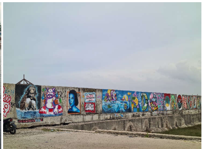
Figure 5. The eastern seawall covered in artistic graffiti representing the theme of sinking.
