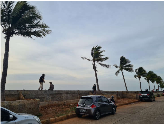
Figure 14. The western seawall.
