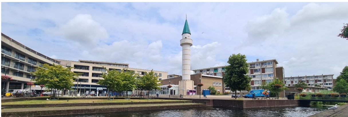
Fig. 7: The Kooiplein (left) and the Imar Sinan Mosque (right) from the back. The room where the activity took place was on this side of the mosque (in white), the entrance was on the other side of the building.
