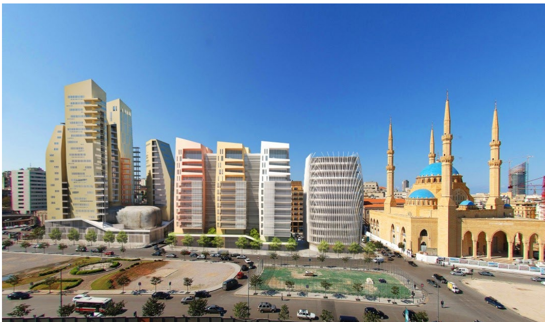
Figure 5.5. Christian de Portzamparc’s architectural design called ‘non construit’ for the Egg and its surrounding area. Source: Christian Deportzamparc Website.
