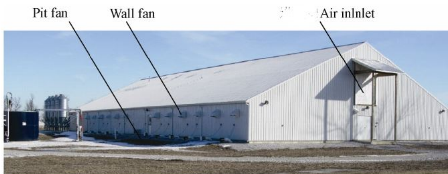
Figure 2: Photo of the pig building, reprinted from Xie et al. (2017) [43, Figure 3a]
