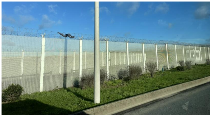
Figure 1: Donnaint, F. (2023). Fences installed along the highway near the port.
