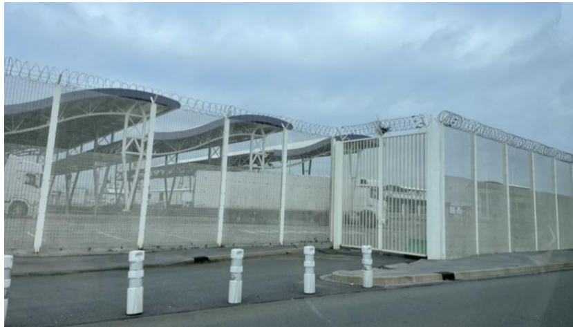
Figure 2: Donnaint, F. (2023). Fences installed along the highway near the port.
