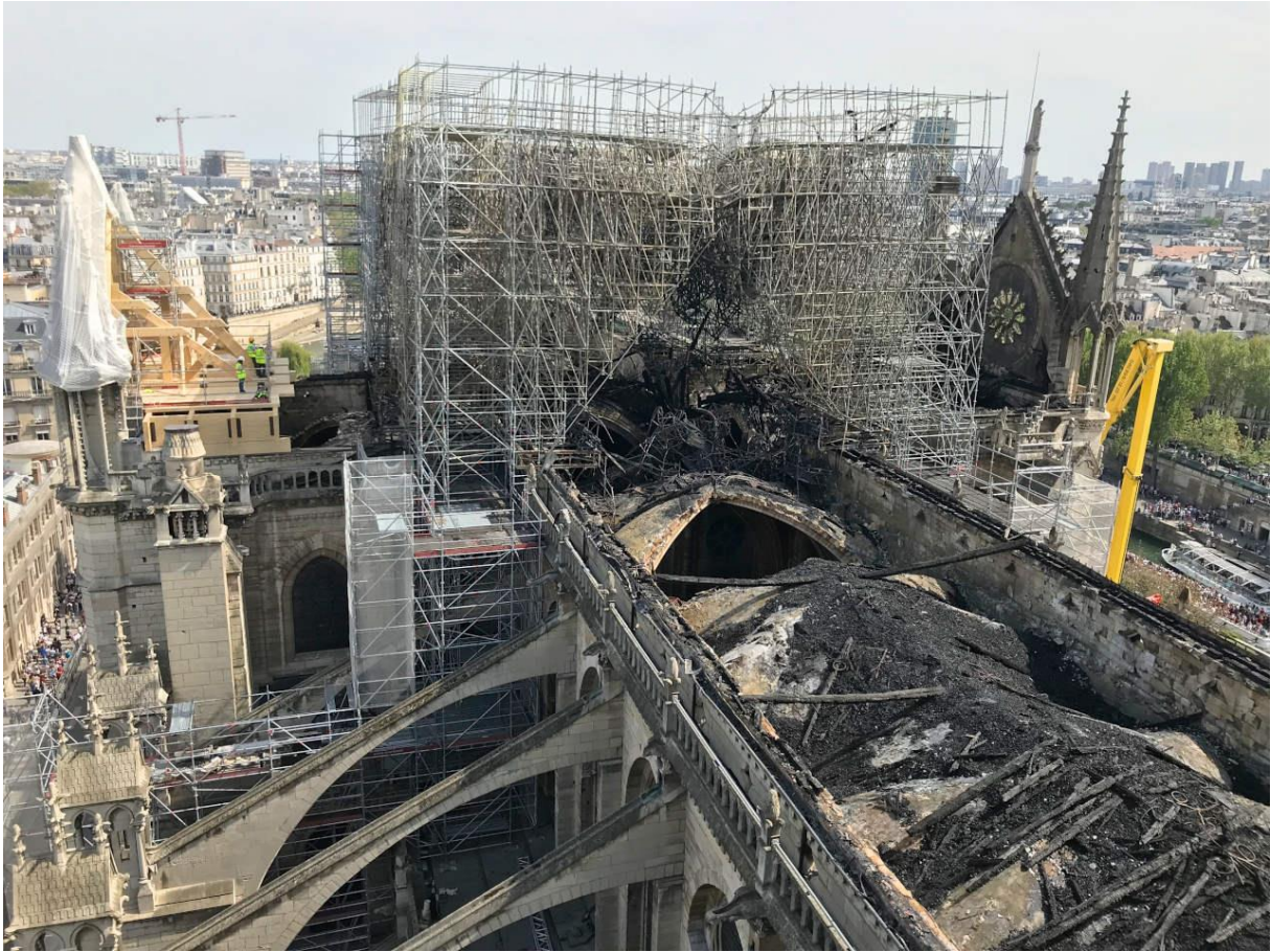
Figure 4.3. The roof of the Notre-Dame after the firefighters had stopped the fire. Source: Friends of Notre-Dame de Paris.
