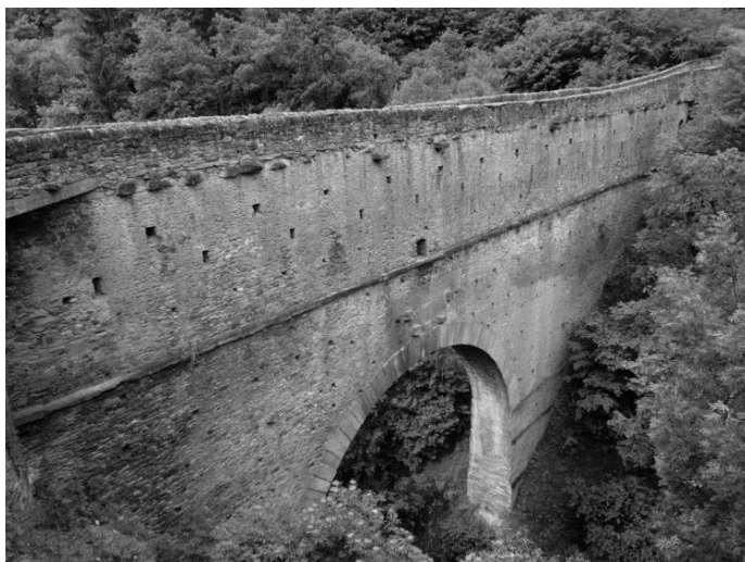
Figure 23. Pondera aqueduct bridge, Italy (Willi, 2019, p.78)
