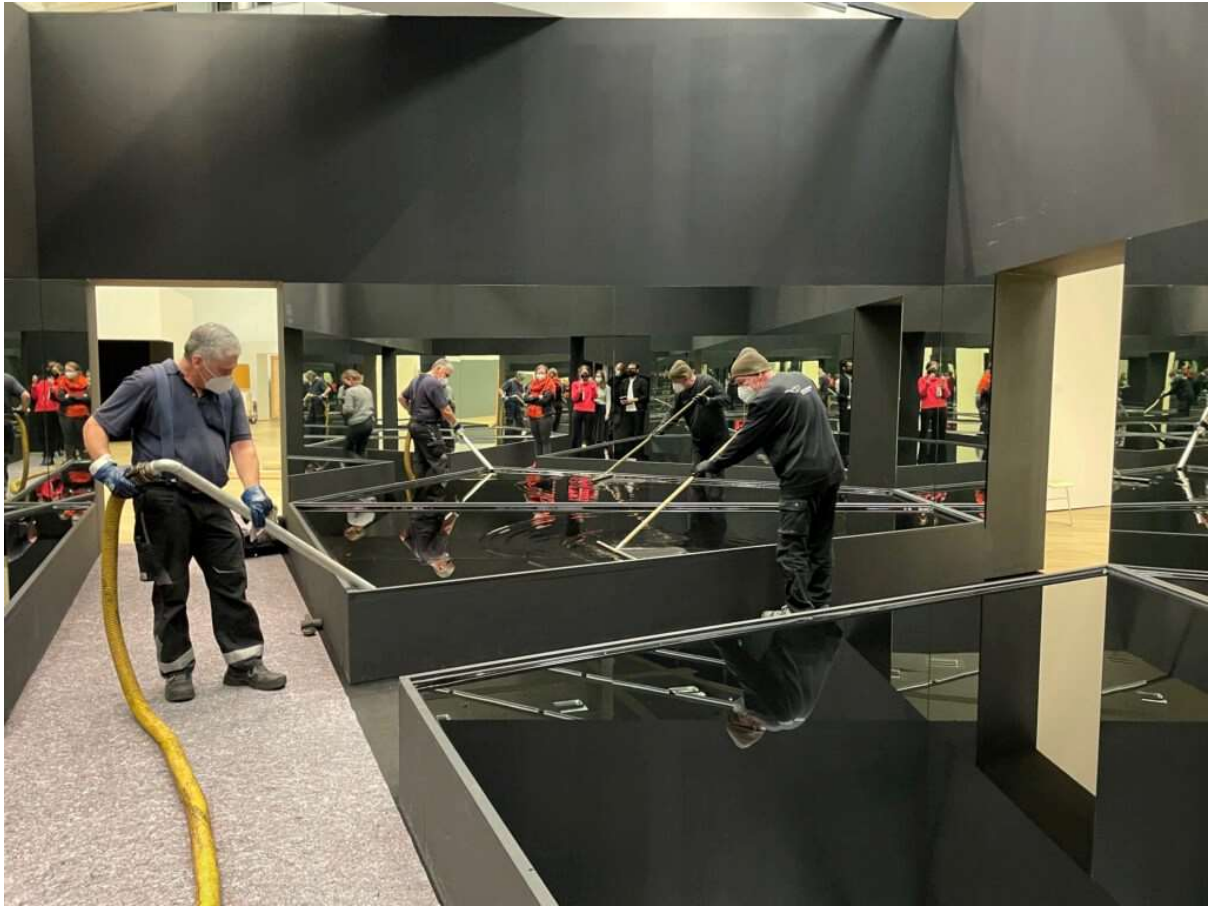
Image 9: The dismantling of the art installation Ölspiegel, pumping and cleaning the vessels of oil.
