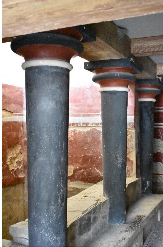
Figure D13 View of the lustral basin from northeast, with the restored columns and the decoration of the south wall visible. South space of the main room in the Throne Room complex, palatial complex of Knossos. Detail of the image used for the reconstruction of the wall decoration in 3D by the author. (Figure: V. Georgiopoulou).
