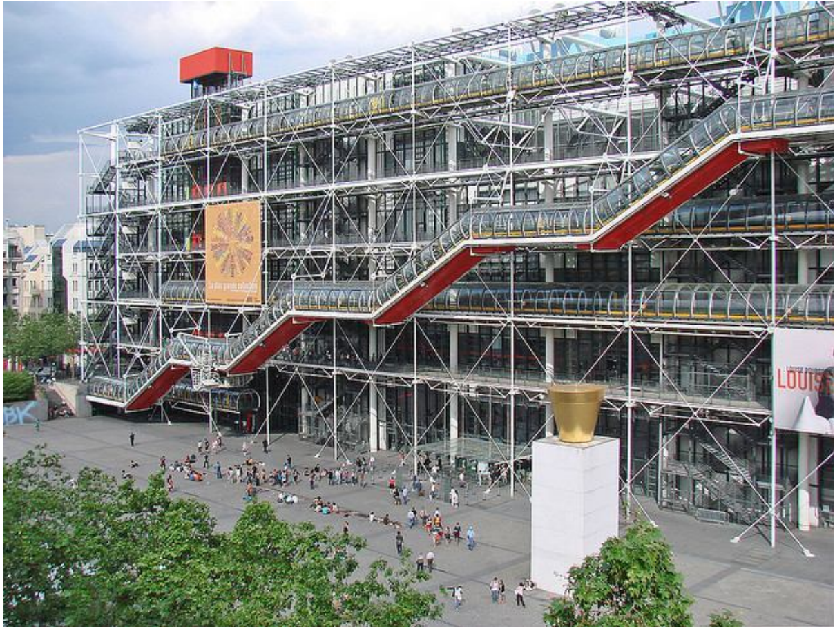
Fig. 33: Paris, Centre Pompidou building , 1977, Renzo Piano & Richard Rogers, collection building of the Musée national d'art modern. Photograph by dalbera.
